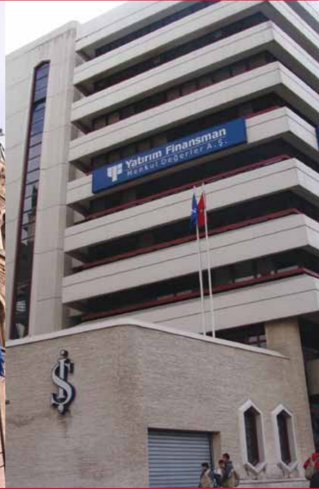
ANKARA KIZILAY OFFICE BUILDING
